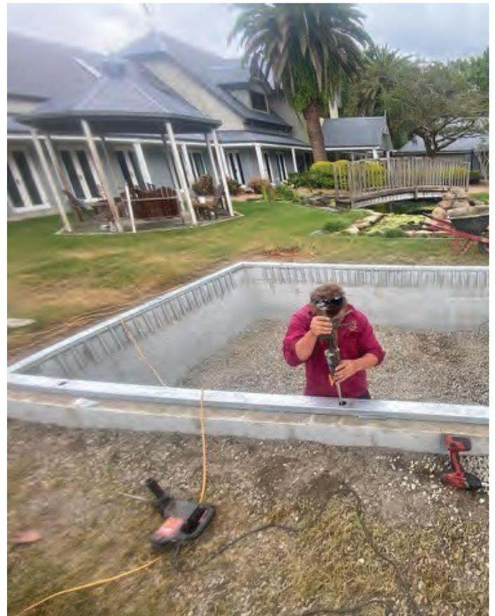
*Tradesman in action bolting down the frame to the masonry walls of the pit.*
